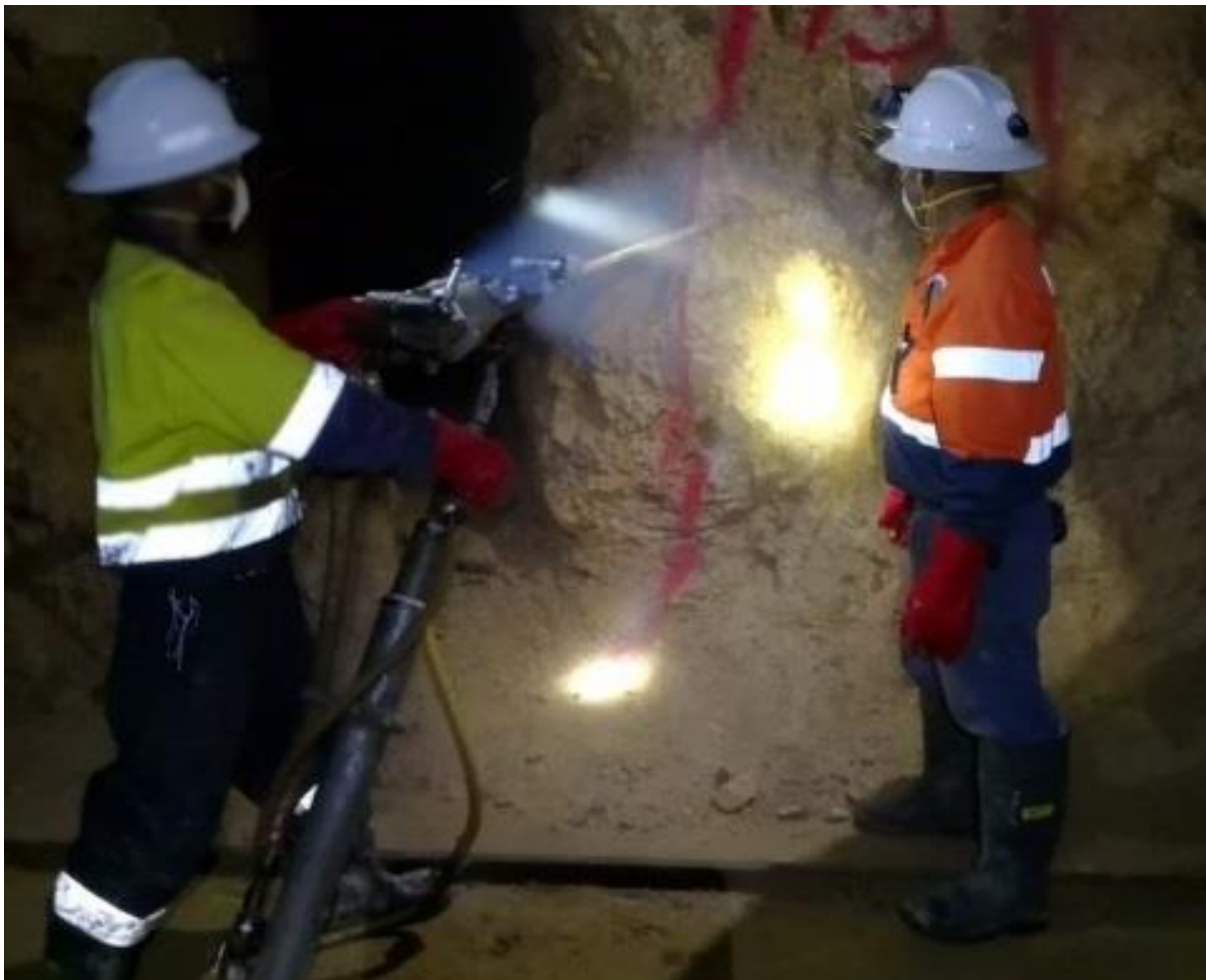
Photo 1: commencement of Gold Mining at HGZ Project, Crater Mountain.
