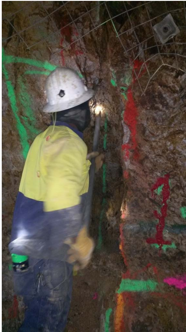
Figure 1 - Face preparation NV1 drive, one of the three veins currently being developed
