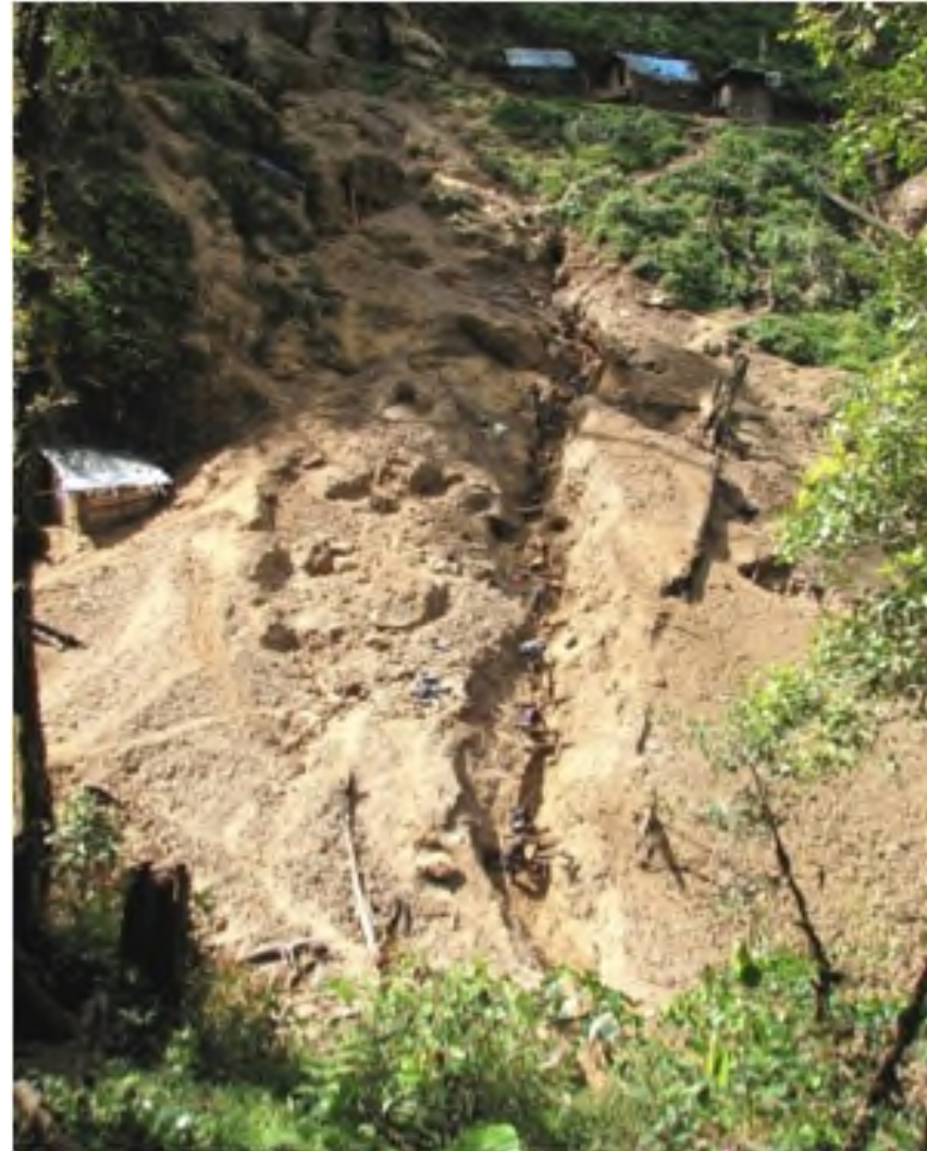
Sluice boxes in gutter in scree below hardrock workings
